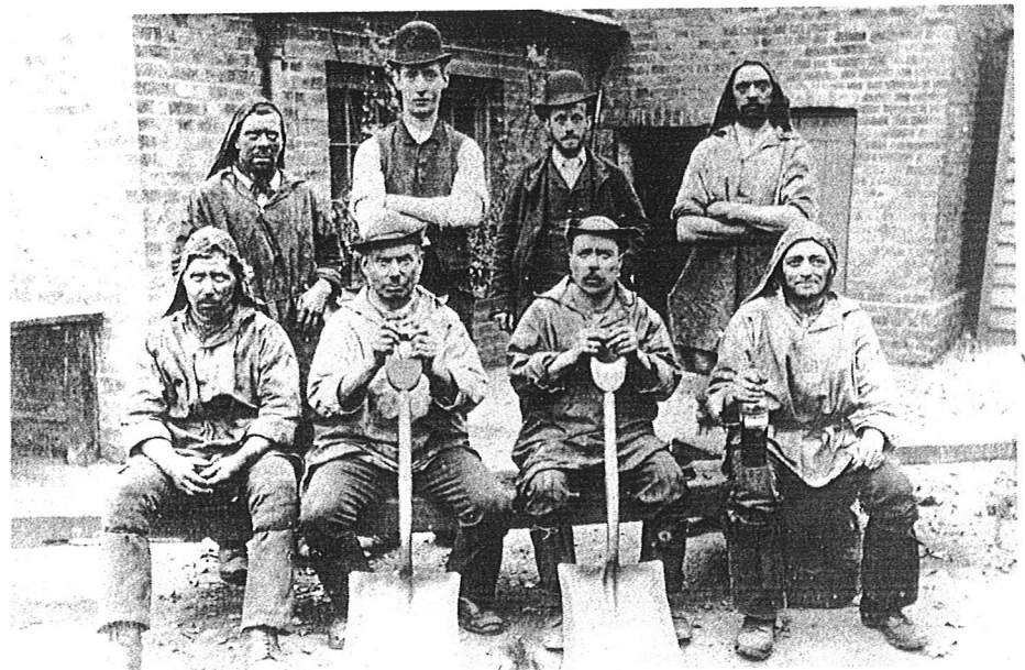
The boiler house gang. Four of the men have head coverings for protection when carrying coal. Two others have large shovels, which leaves the foreman and chargehand in their bowler hats.
