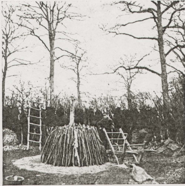
FIG. 12. 'CORDWOOD' BEING PILED ON 'COAL-HEARTH' BEFORE BURNING (Photographed by Mr. Miller Christy in the Writtle Highwoods)
