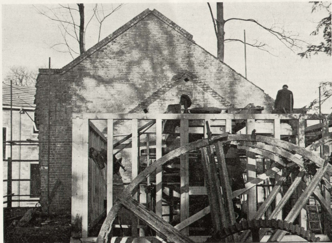
Chart Mills : surviving mill in course of restoration, April 1969
