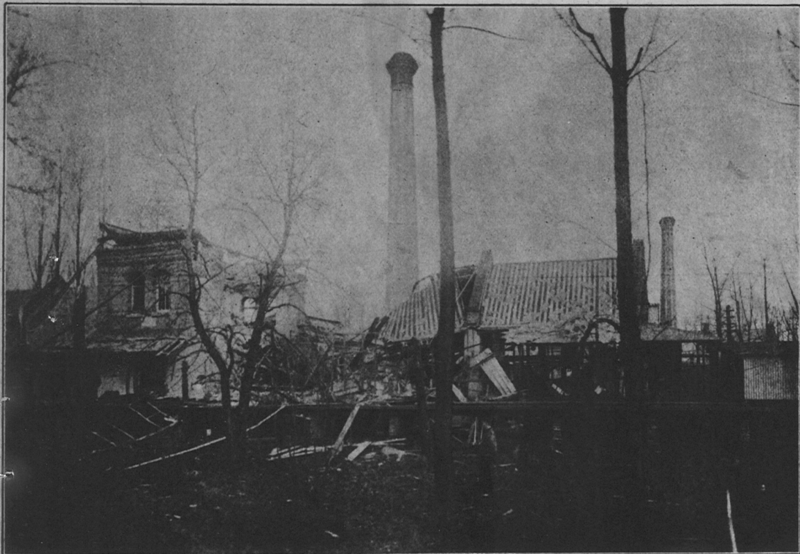
ENGINE HOUSE AND BAYS 3, 2, 1, GROUP G.
