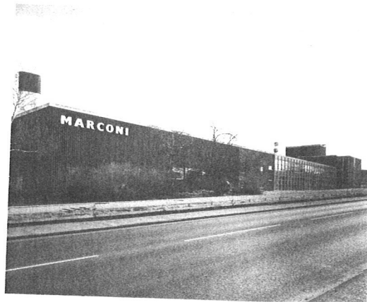
Figure 13. Marconi, Waterhouse Lane, Chelmsford. Its position on ring road is typical of many post-war electronics factories, as is the high proportion of the building given over to technical design and administrative functions compared to assembly activities (AA99/01821 © Crown copyright. NMR).
