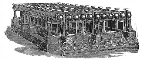
10. Series of 22 cast-iron pipes about 11 ft long for heating 256 trays which could dry 30 to 40 barrels of gunpowder. The small pipes in the foreground are for draining away condensed steam. Constructed by Taylor & Challen of Birmingham: from *Engineering* of 1878.
