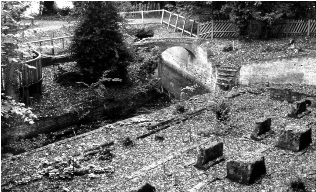
Site of glazing house, late 19 th century and refurbished in 1926 (W D Cocroft)
