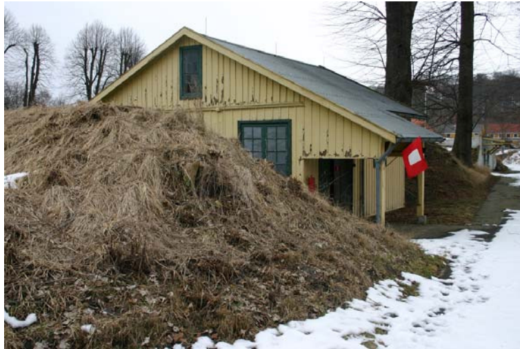
The Sorting House partly hidden behind earth rampart. The flag shows that a machine is running.
