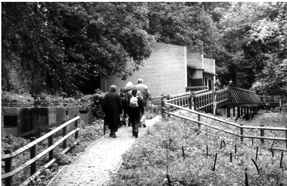
The part restored 1926 gunpowder incorporating mill with mill bay and motor room (W D Cocroft)
