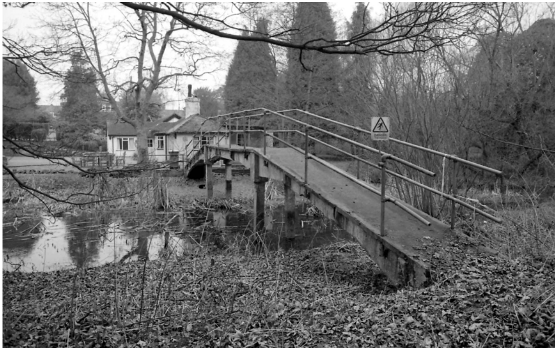
Footbridge and watch house (W D Cocroft)
