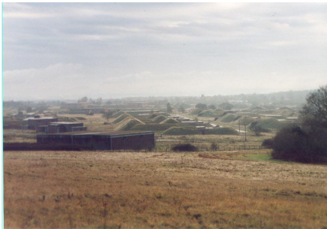
View looking east over Press Houses Unit 2
