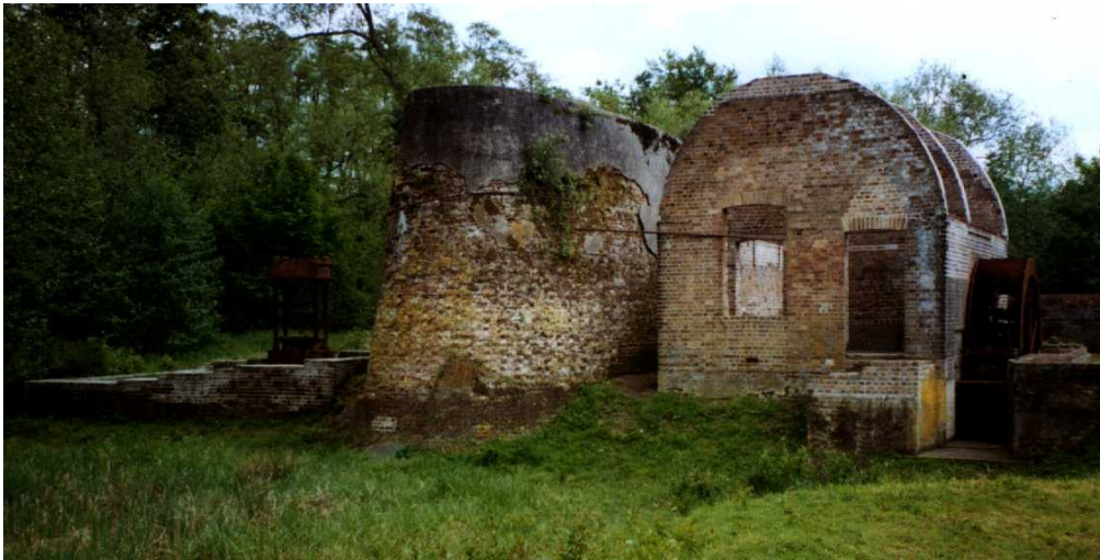
The Presshouse - to the right is the waterwheel and pumphouse, in the centre is the traverse and the left is the gunpowder press.
