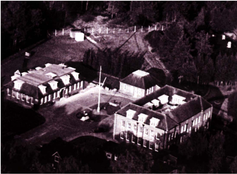
RNCF Holton Heath, the main administration buildings, courtesy of the RNCFA
